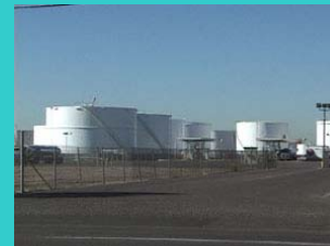
7. Ethanol unloaded from tank trucks for storage separately from gasoline
